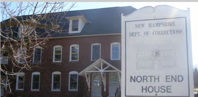
North End Transitional Housing Unit (C1)
