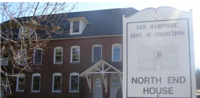
North End Transitional Housing Unit (C1)
