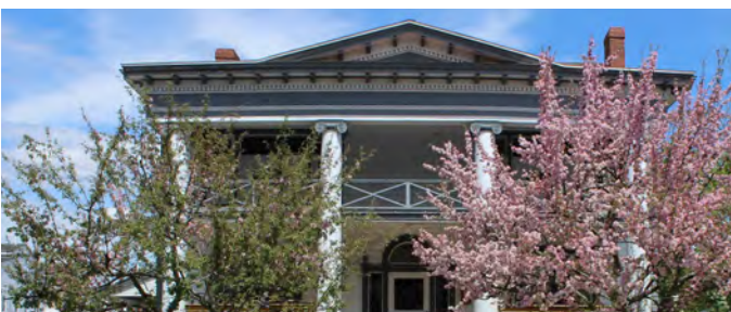
Calumet Transitional Housing Unit (C1)
